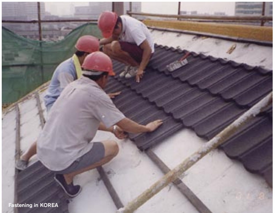
Using wooden packers
