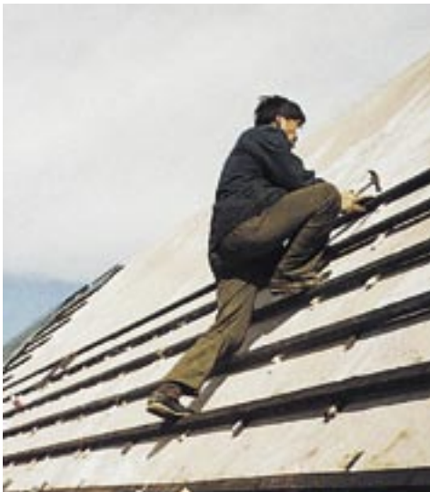
Installation in progress, Hu Tan Park, Dalian, CHINA
