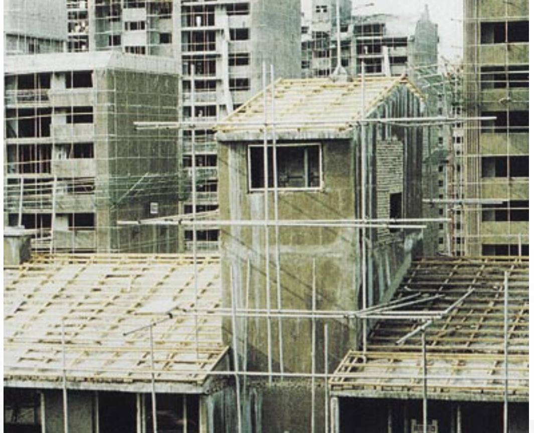
ABOVE: Installation in progress, using counter batten system, Boondang Apartments, KOREA
